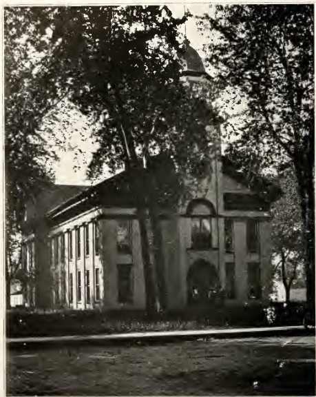
POWESHIEK COUNTY COURTHOUSE
